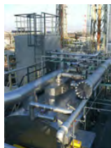
Sludge dryer system (Yokkaichi Plant)
