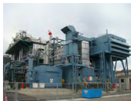
Natural gas-fired turbine cogeneration system (Yokkaichi Plant)
